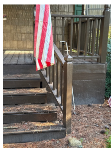
2.3 Item 1 (Picture) Front exterior
