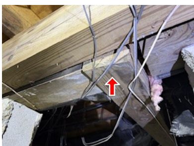
5.0 Item 12 (Picture) Rear of crawl
