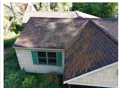
1.0 Item 3 (Picture) View of roof
