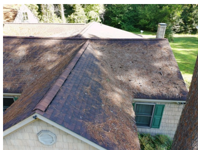
1.0 Item 1 (Picture) View of roof
