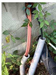
7.3 Item 1 (Picture) Rear right exterior
