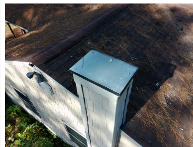
1.0 Item 6 (Picture) View of roof
