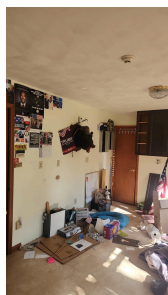
7.3 Item 2 (Picture) detached garage office room outlets
