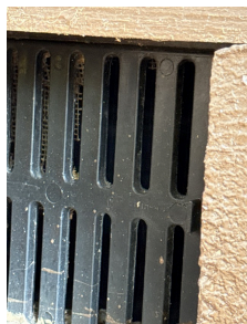
5.0 Item 1 (Picture) Front exterior
