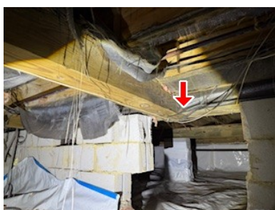
5.0 Item 13 (Picture) Rear of crawl
