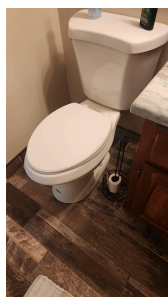
6.0 Item 1 (Picture) hallway bathroom toilet
