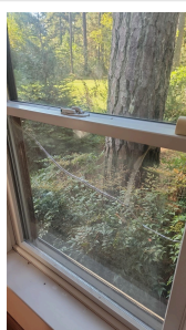
2.2 Item 1 (Picture) front right bedroom front window
