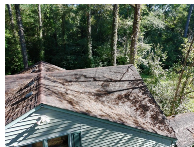
1.0 Item 9 (Picture) View of roof
