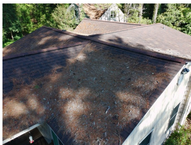
1.0 Item 5 (Picture) View of roof
