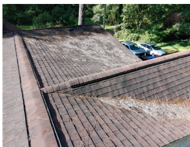
1.0 Item 2 (Picture) View of roof
