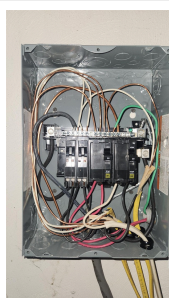
7.1 Item 1 (Picture) detached garage rear right wall
