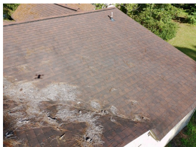
1.0 Item 4 (Picture) View of roof
