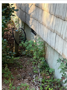
2.4 Item 5 (Picture) Right exterior
