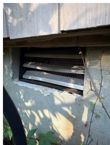
5.0 Item 3 (Picture) Right exterior
