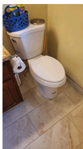
6.0 Item 2 (Picture) primary bathroom toilet
