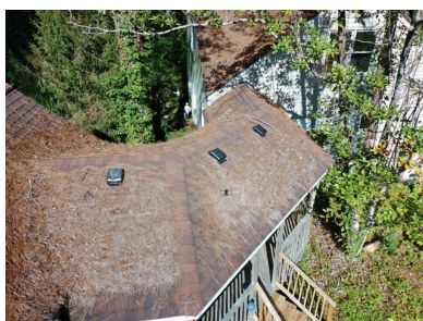
1.0 Item 8 (Picture) View of roof
