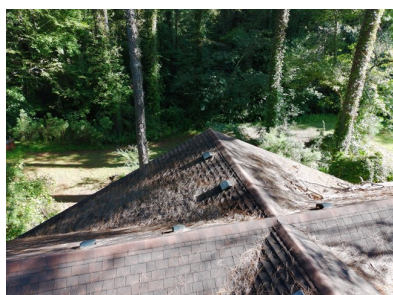
1.0 Item 7 (Picture) View of roof
