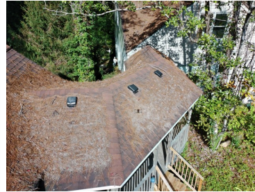
1.0 Item 8 (Picture) View of roof
