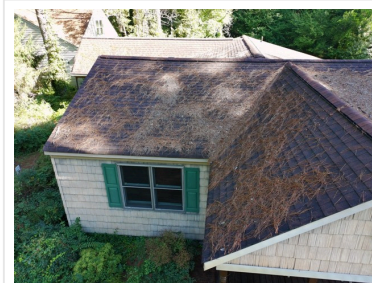
1.0 Item 3 (Picture) View of roof
