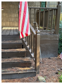
2.3 Item 1 (Picture) Front exterior
