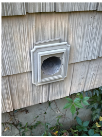
2.0 Item 4 (Picture) Rear exterior
