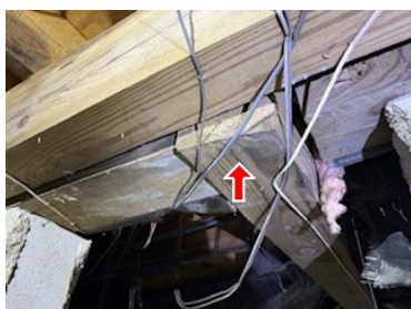
5.0 Item 12 (Picture) Rear of crawl
