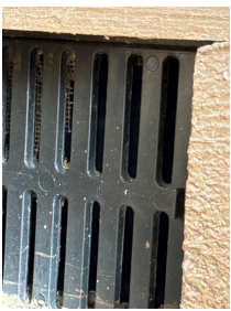
5.0 Item 1 (Picture) Front exterior
