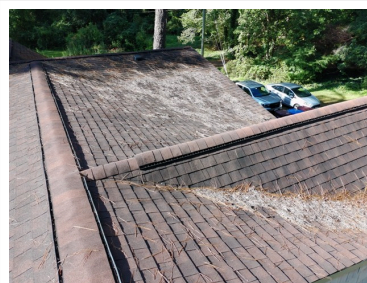
1.0 Item 2 (Picture) View of roof
