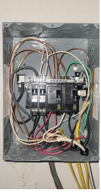
7.1 Item 1 (Picture) detached garage rear right wall
