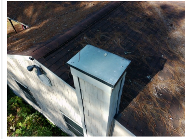
1.0 Item 6 (Picture) View of roof
