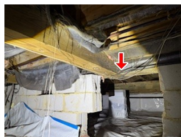
5.0 Item 13 (Picture) Rear of crawl
