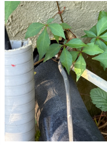
2.0 Item 3 (Picture) Rear right
