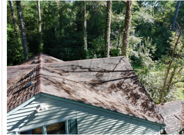
1.0 Item 9 (Picture) View of roof
