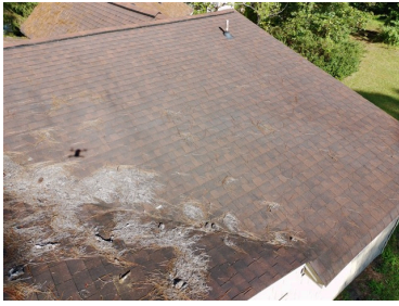
1.0 Item 4 (Picture) View of roof
