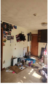
7.3 Item 2 (Picture) detached garage office room outlets
