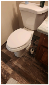
6.0 Item 1 (Picture) hallway bathroom toilet
