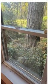
2.2 Item 1 (Picture) front right bedroom front window
