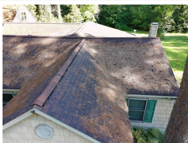
1.0 Item 1 (Picture) View of roof
