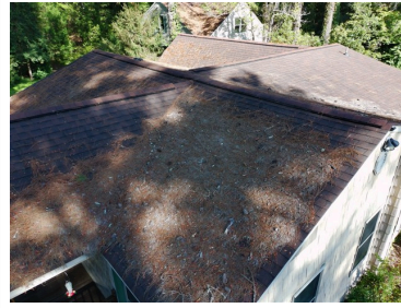
1.0 Item 5 (Picture) View of roof
