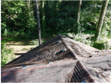
1.0 Item 7 (Picture) View of roof
